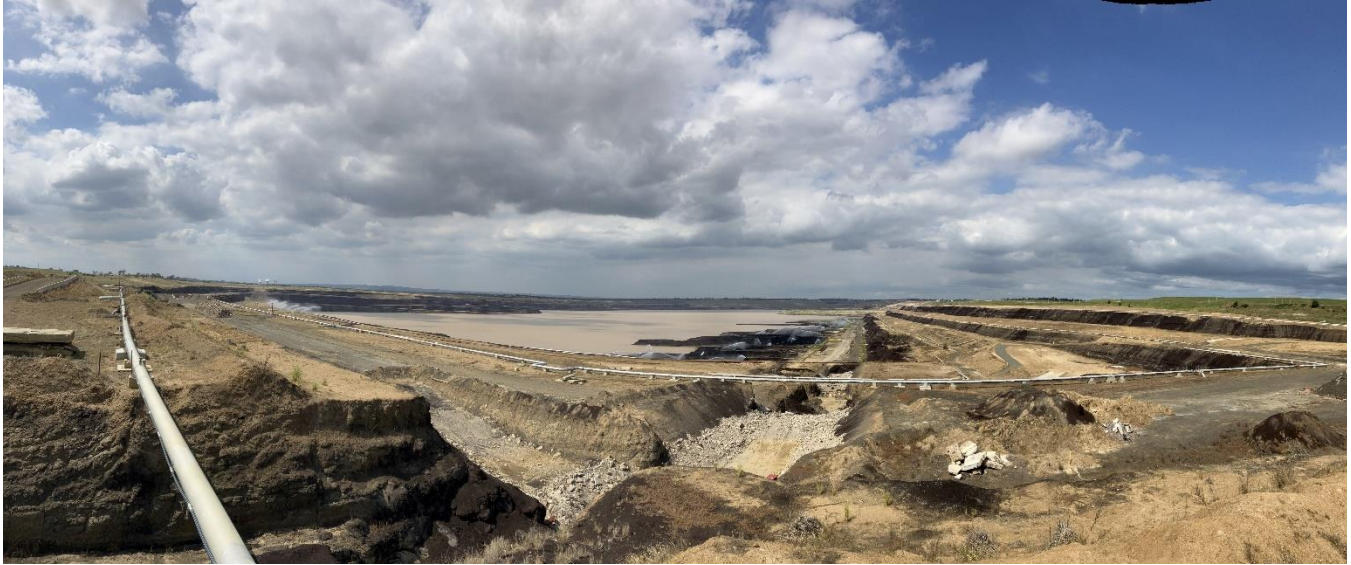
Figure 1: Hazelwood mine void in November 2023
