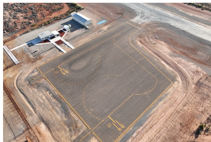
Upgraded Kambalda aerodrome, photograph courtesy of the Shire of Coolgardie
