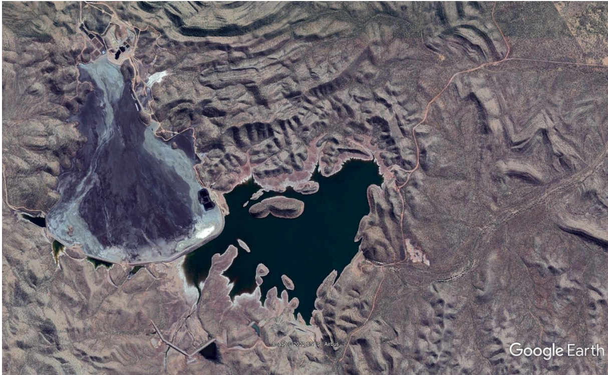
Figure 27: Google Earth image of Century Zinc Mine tailings storage facility (June 2018)
