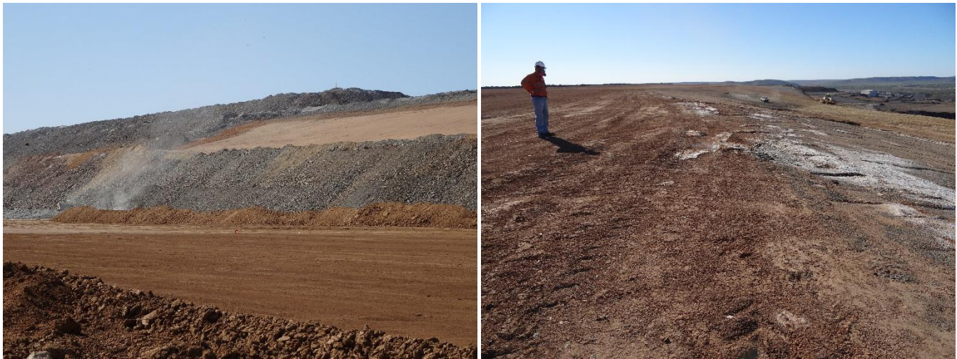
Figure 36: Breakthrough of a compacted rock layer due to spontaneous combustion of thinly-covered sulfidic waste rock
