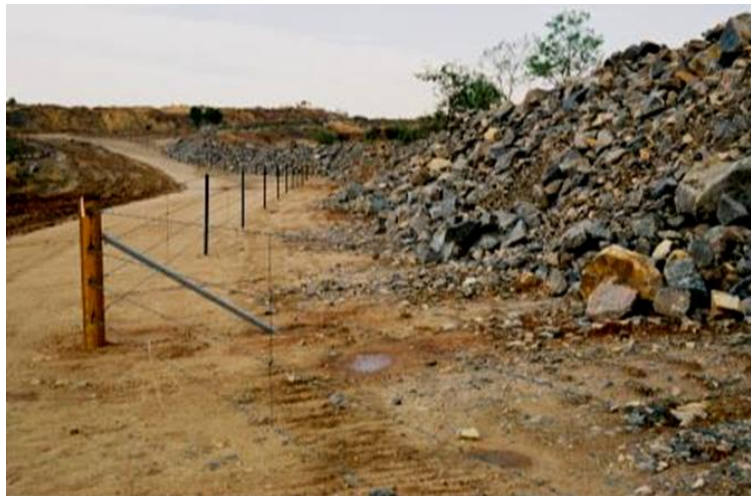
Figure 6: Bunding and fencing around crest of a closed open pit
