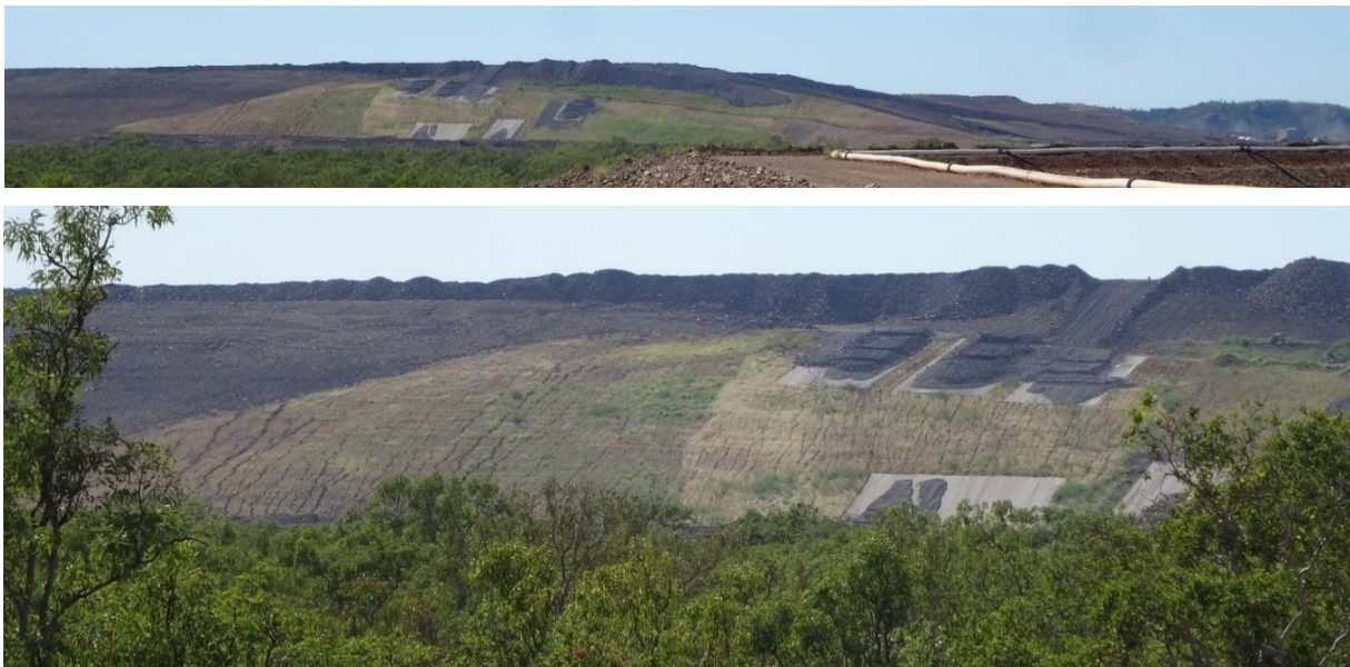
Figure 43: Progressive rehabilitation of North Overburden Emplacement Facility in accordance with Supplementary Environmental Impact Statement in April 2021
