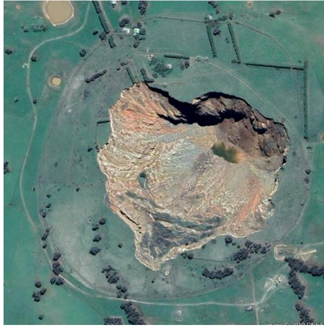
Figure 8: Unrehabilitated block cave
