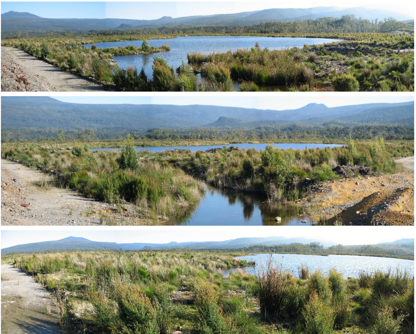
Figure 53: Photographs of peat and water cover over old tailings storage facility at Henty Gold the Google Earth images of Henty Gold Mine tailings storage facilities taken in April 2008
