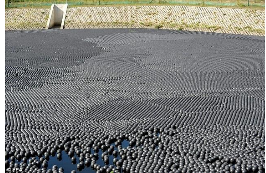
Shade balls on a small reservoir.
