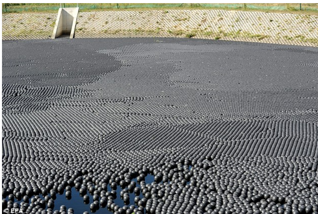
Figure 13: Shade balls on a small reservoir. Image from https://energyvulture.com/2016/02/14/shade-balls-roll-their-way-into-the-spotlight/
